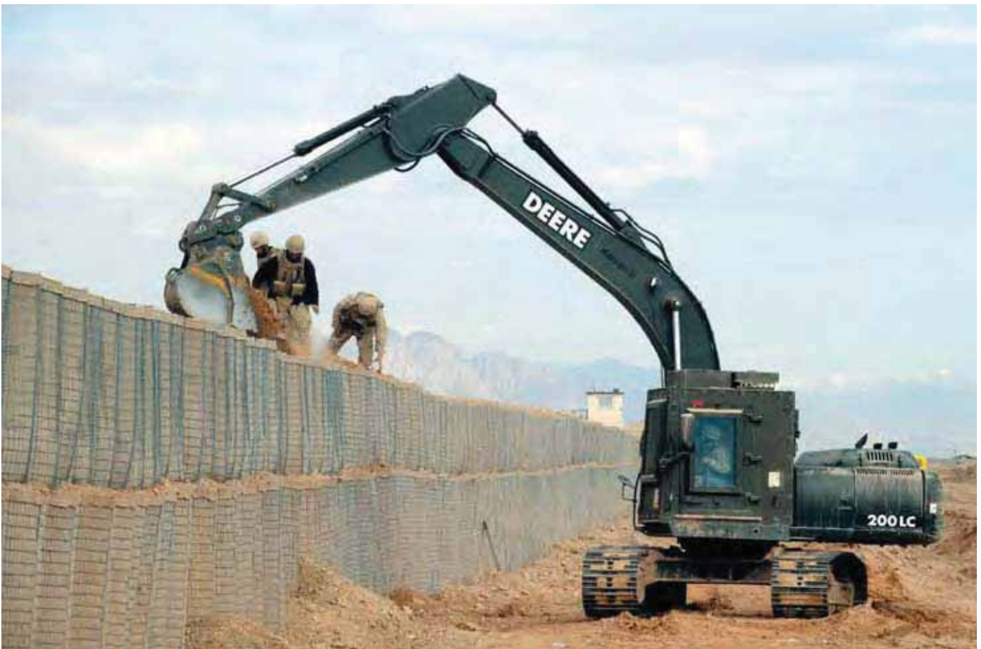
Navy Seabees assigned to Naval Mobile Construction Battalion 7 use an up-armored excavator to fill Hesco barriers at a forward operating base in the Helmand province of Afghanistan Jan. 25. The Defense Logistics Agency began shipping construction materials early this year in anticipation of 17,000 Soldiers and Marines scheduled to deploy there by summer.
